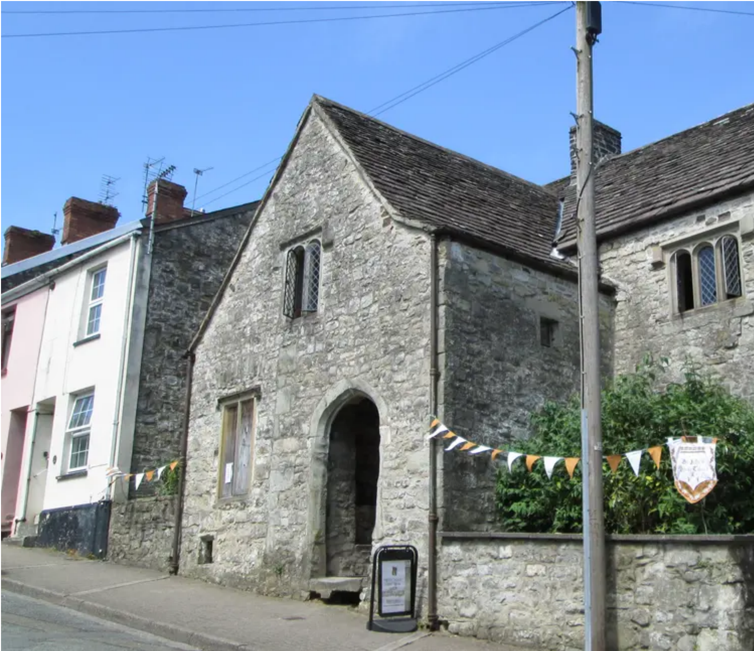
St John's House, Bridgend
