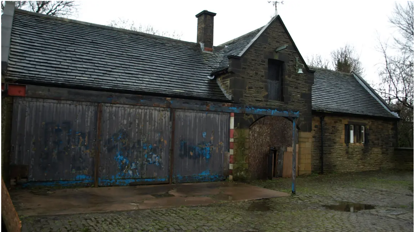
Stables and Motor House at Haworth Art Gallery
