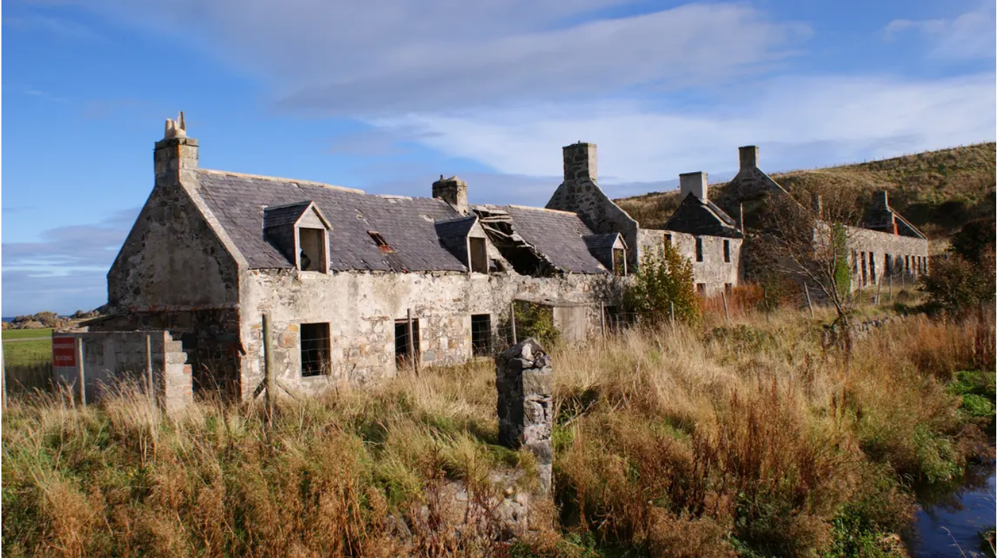
Exterior view of Portsoy Bunkhouse
