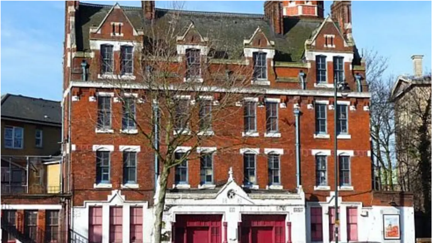
Old Fire Station in West Norwood
