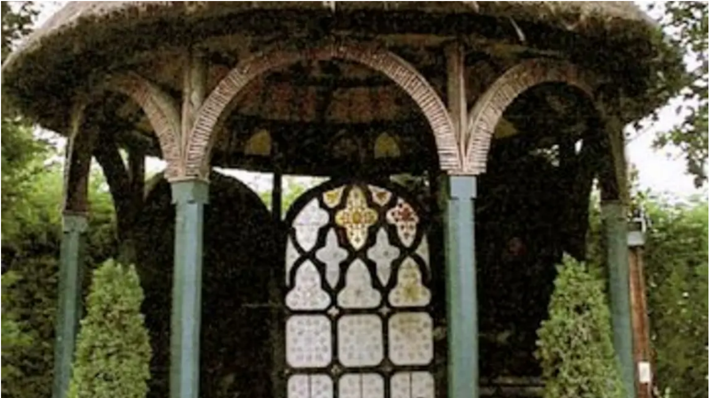
The Grade II* listed Swiss Cottage at the Swiss Gardens, Bedfordshire
