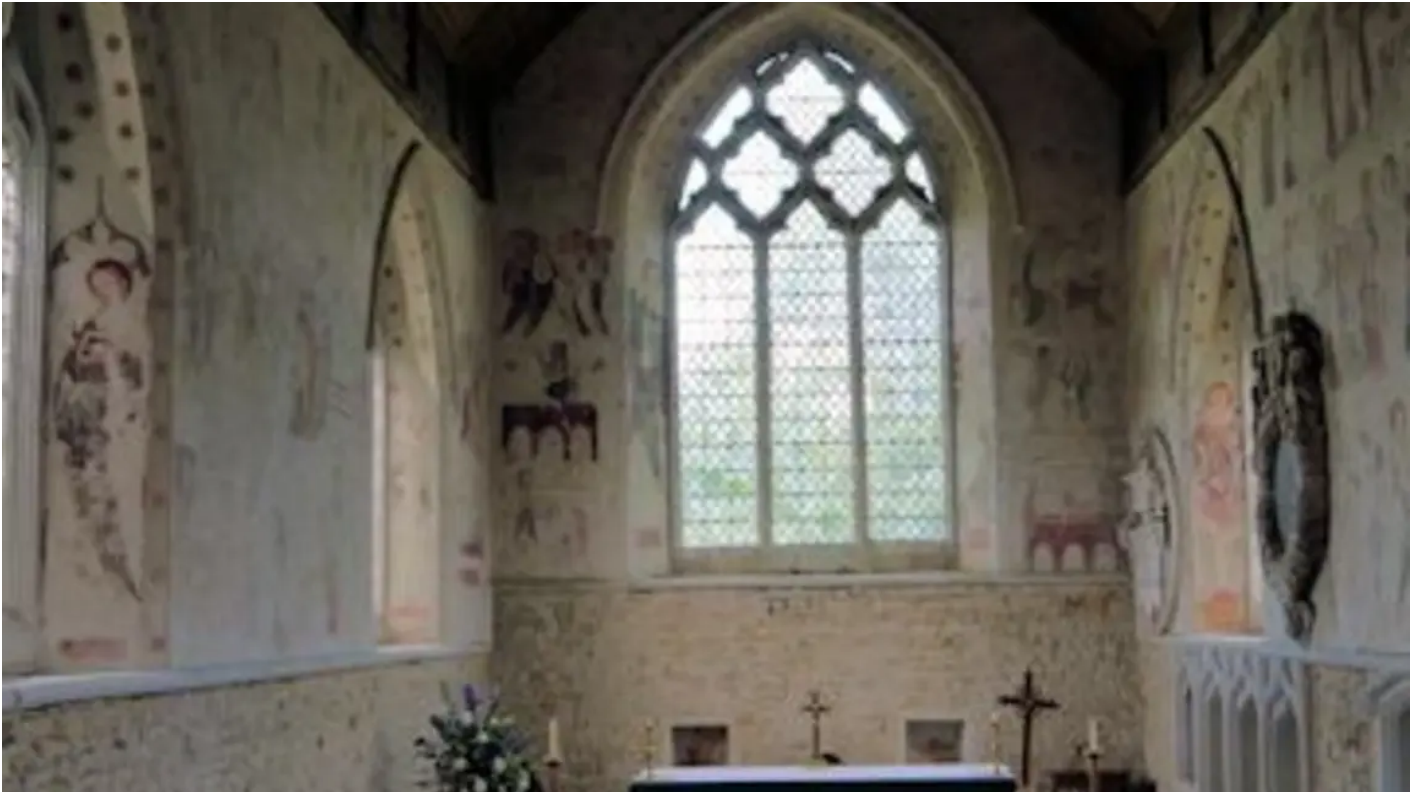
Wall paintings in St Marys Chalgrove will be saved
