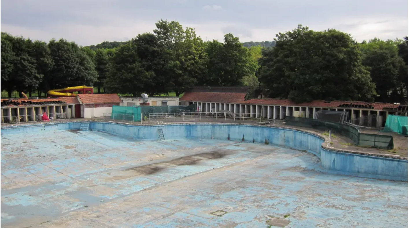
Current condition of Ynysangharad Park Lido
