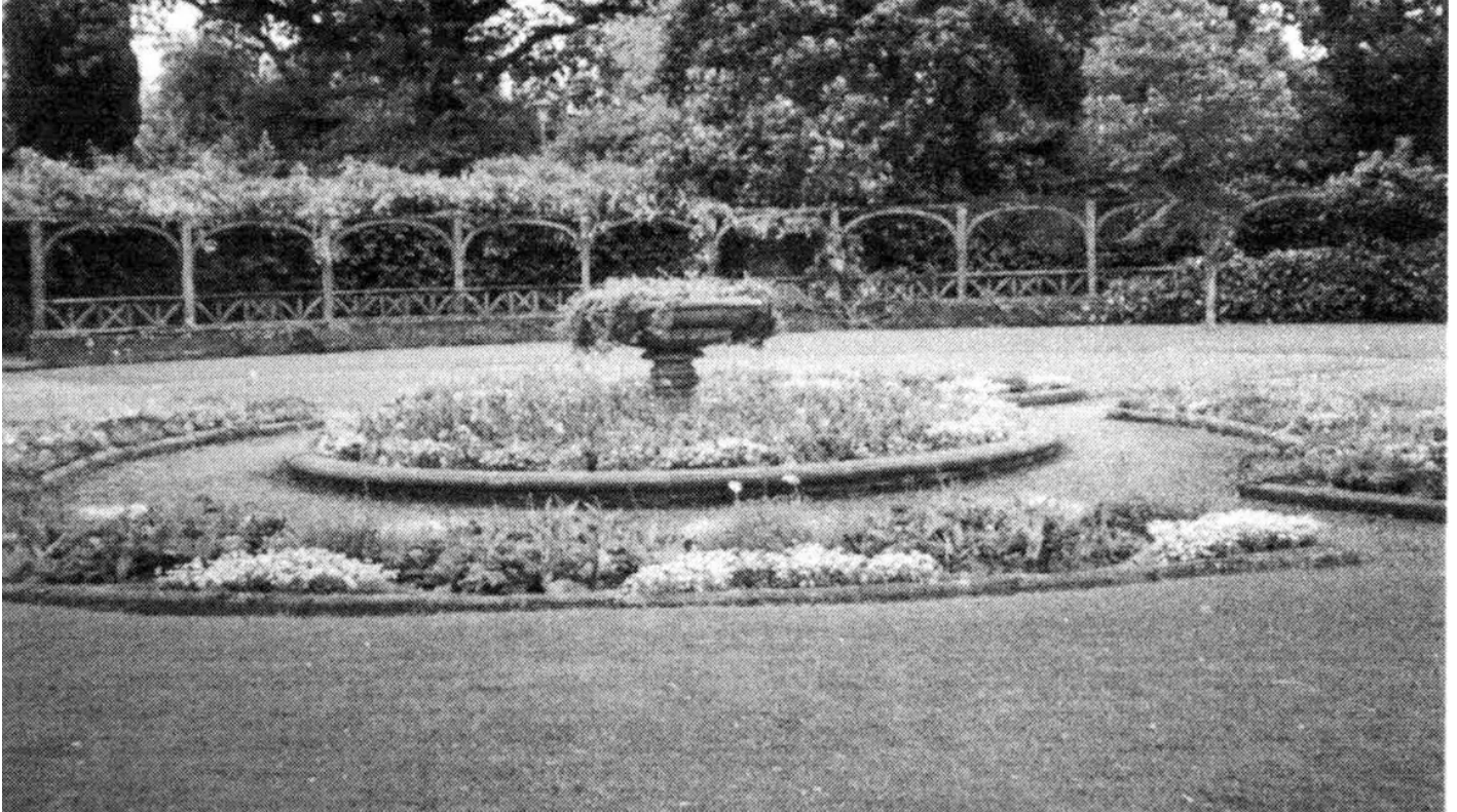
Archive image of the historic Worth Park Fountain Garden
