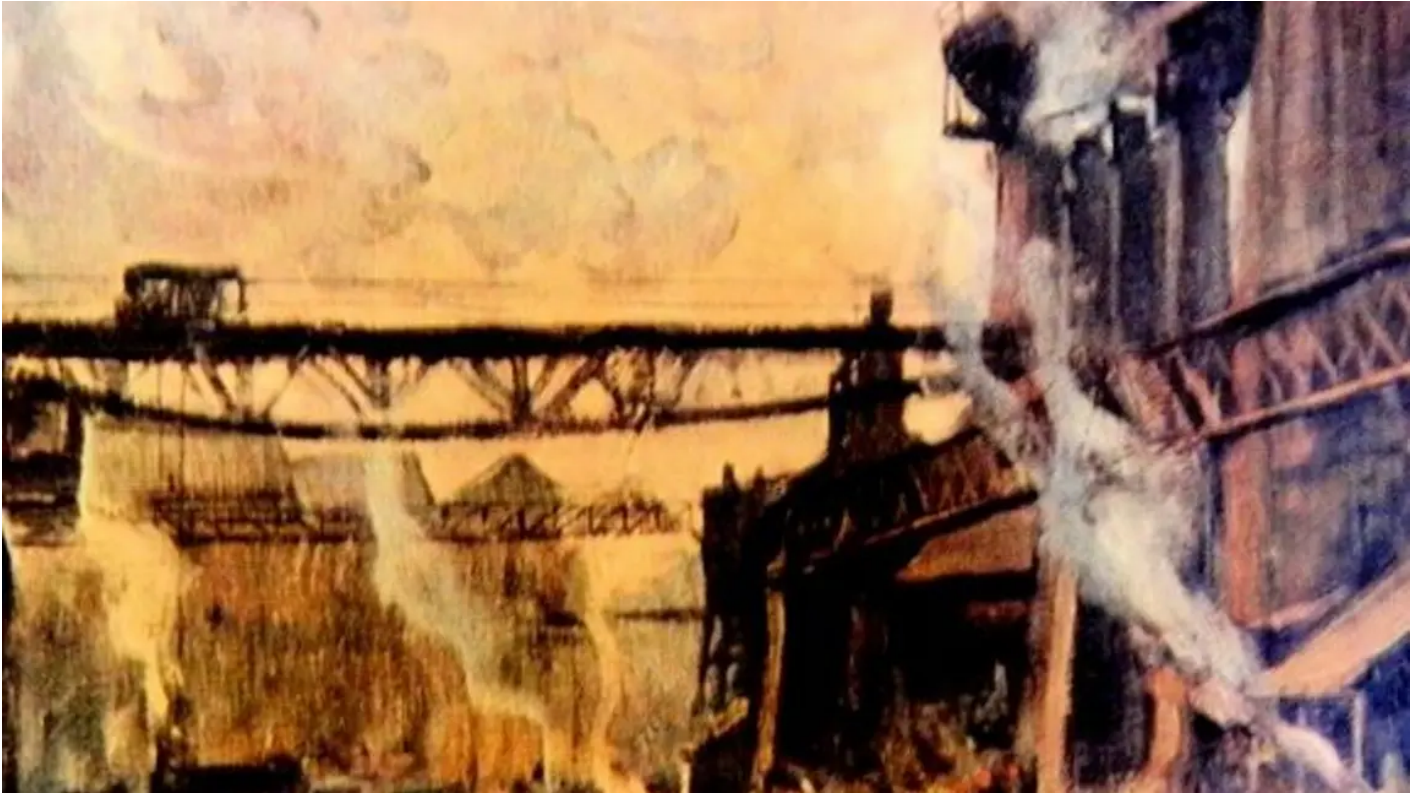
Thorncliffe Blast Furnaces - 1909
