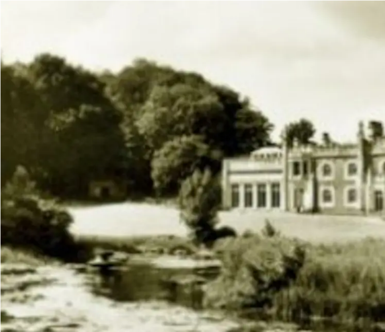
Archive image of the Gothic revival Manor House at Kearsney Abbey
