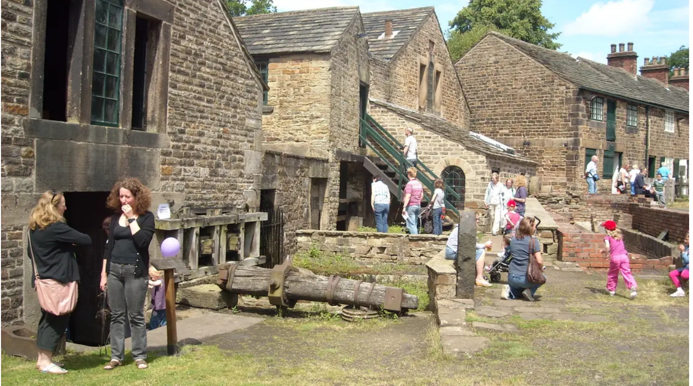
Abbeydale Works part of the Abbeydale Hamlet
