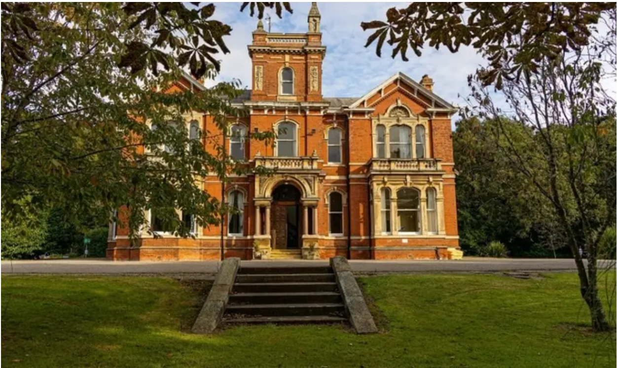
The exterior of Weelsby Hall. Credit: Linkage Community Trust.
