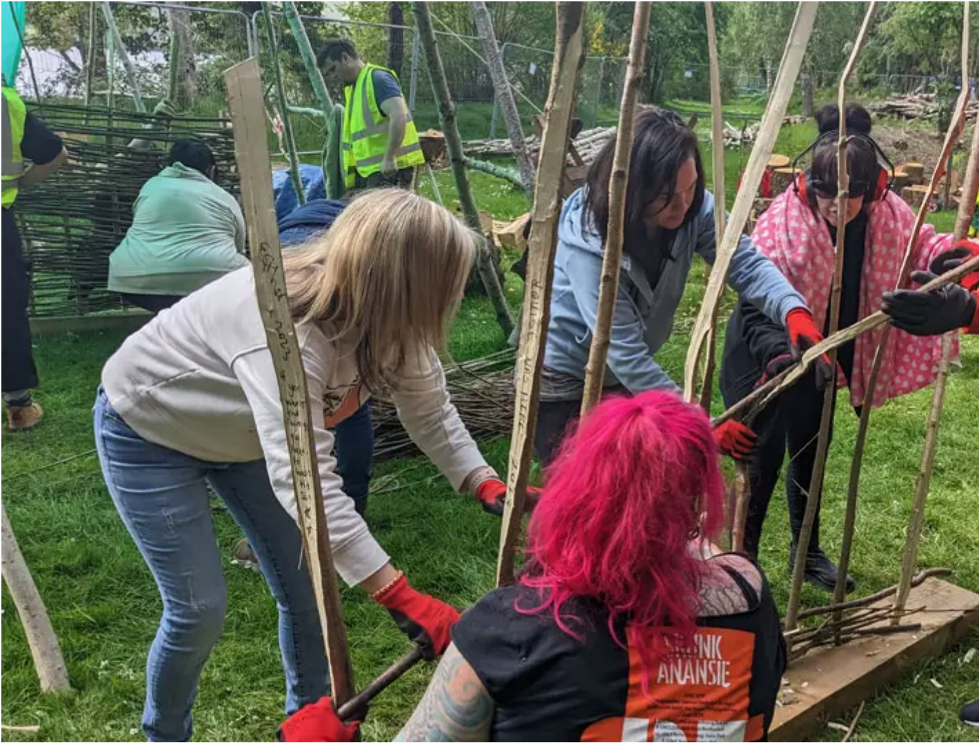
A key component of an Iron Age roundhouse is a basket frame structure for the roof made from hundreds of hazel rods. Photo: The Scottish Crannog Centre.
