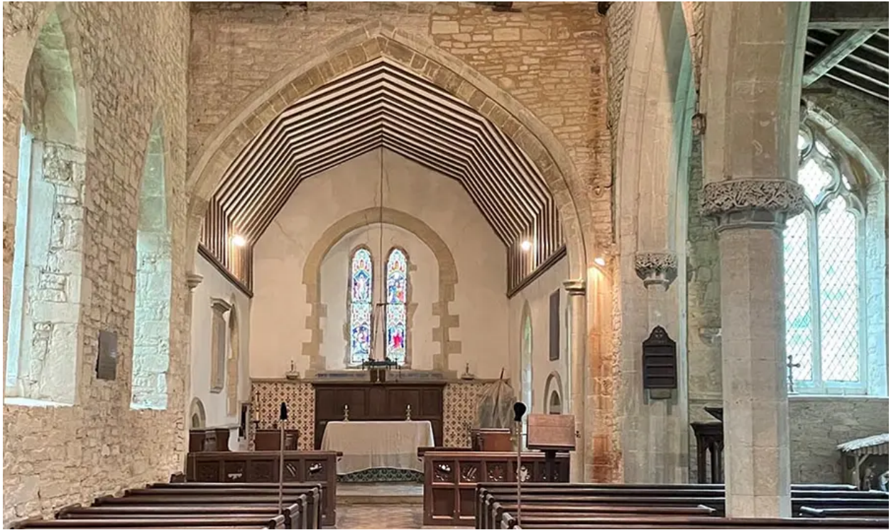
The new ceiling at St Lawrence Church, Radstone.
