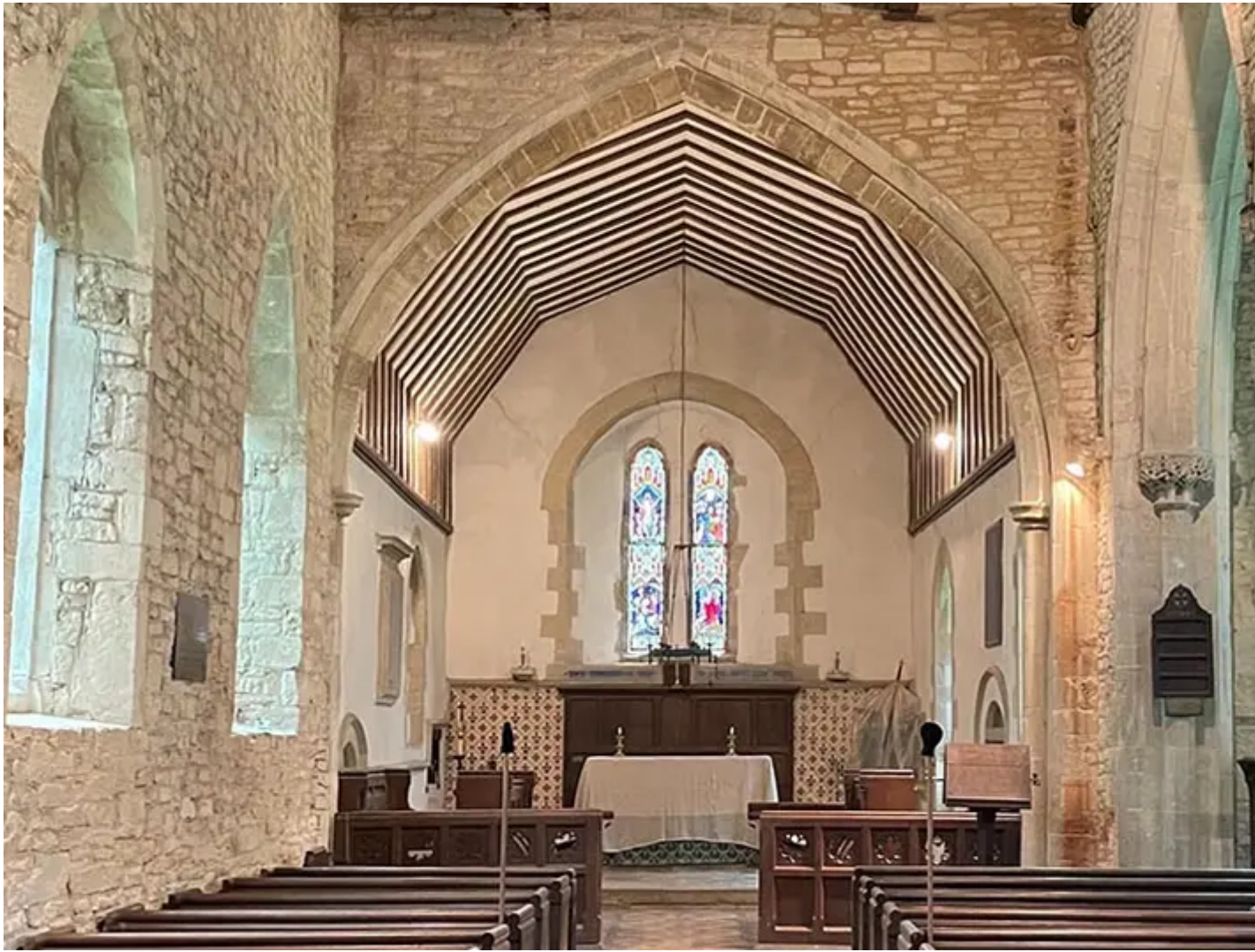
The new ceiling at St Lawrence Church, Radstone.
