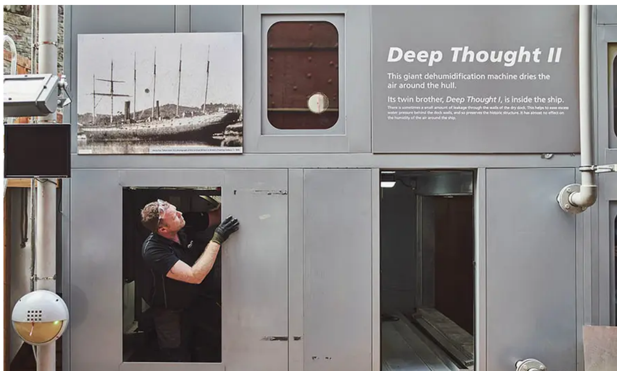
Refitting the dehumidifier fans that preserve SS Great Britain. Photo: Adam Gasson / Munters / SS Great Britain Trust.
