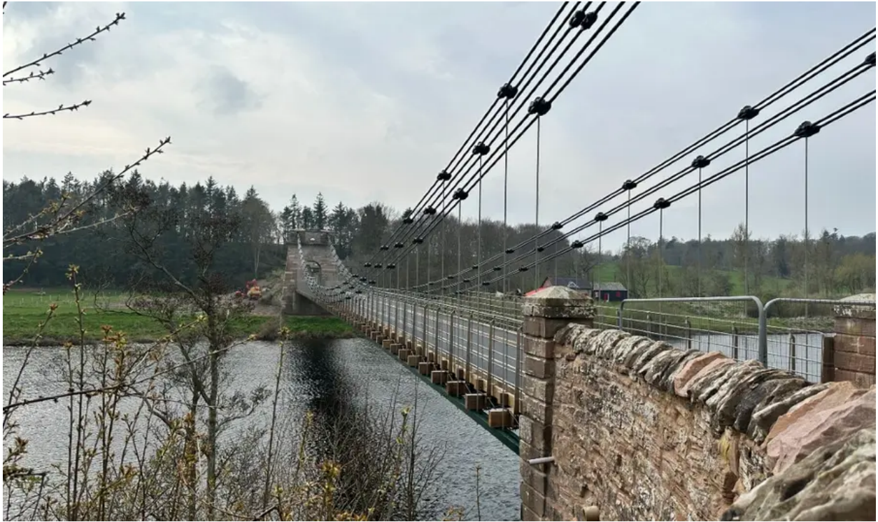
The Union Chain Bridge. Credit: Northumberland County Council
