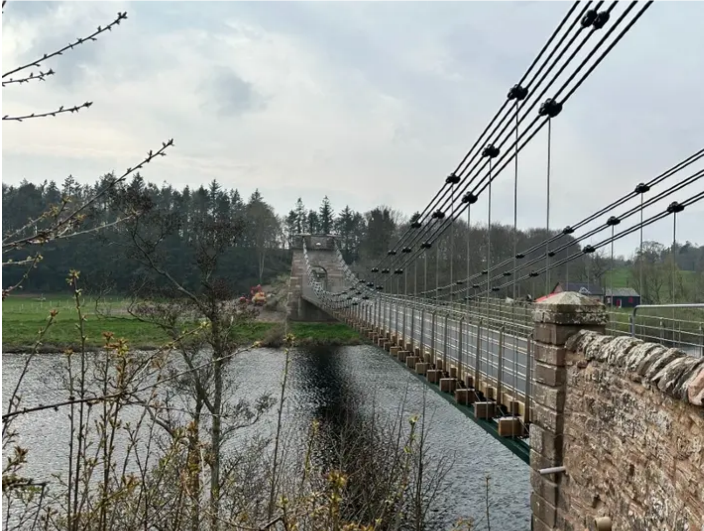
The Union Chain Bridge. Credit: Northumberland County Council
