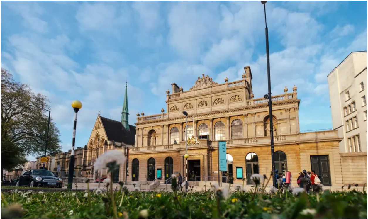
RWA exterior following capital works. Credit: Evan Dawson
