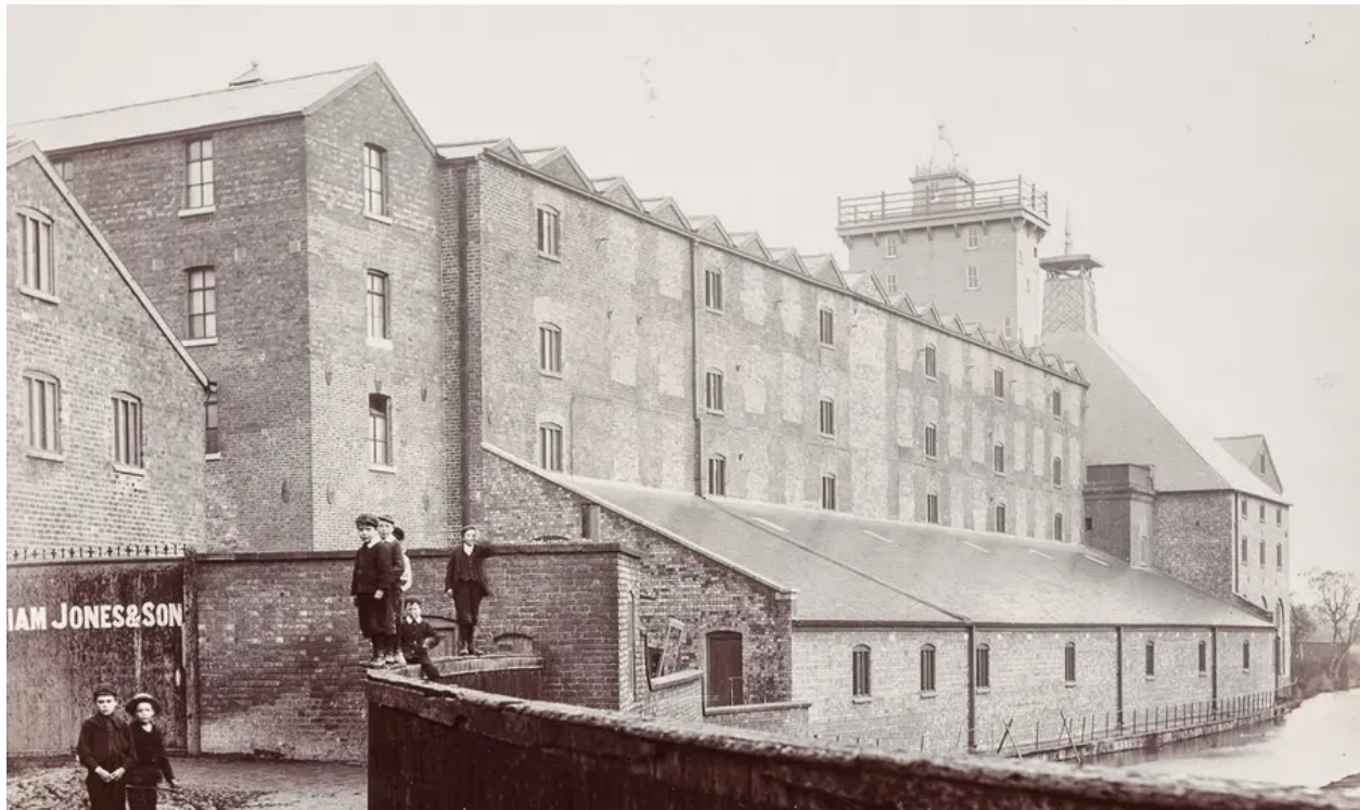
19th century image of the site after it had been adapted for use as a maltings. Credit: Shropshire Archives
