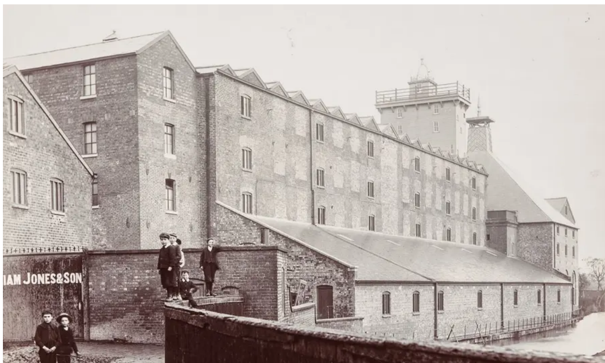
19th century image of the site after it had been adapted for use as a maltings. Credit: Shropshire Archives
