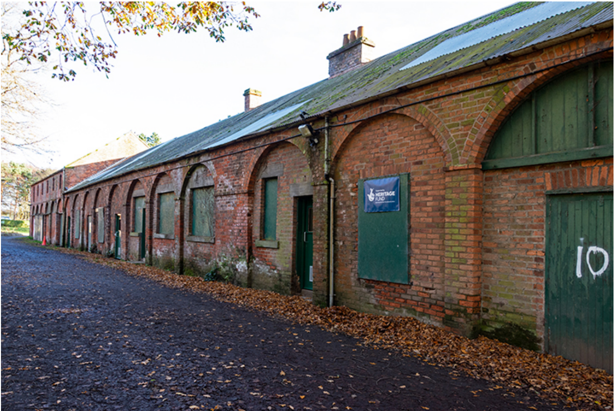
Exterior view of Silverburn Flax Mill
