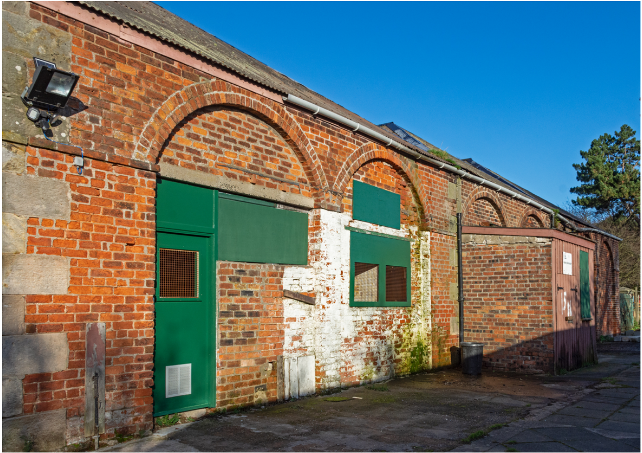
Exterior view of Silverburn Flax Mill
