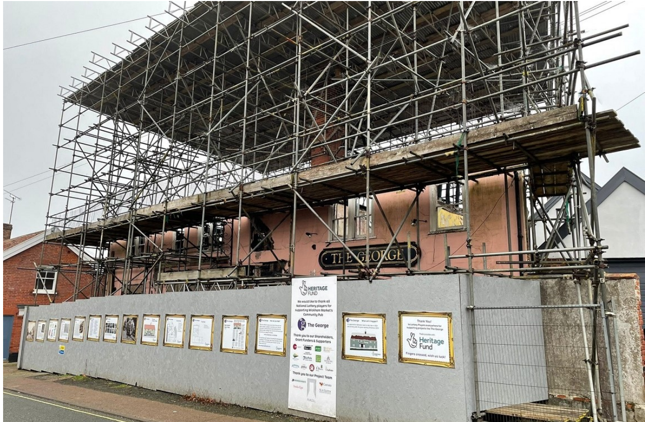
Scaffolding outside the pub to prepare for construction. Credit: Bill Wolff-Evans
