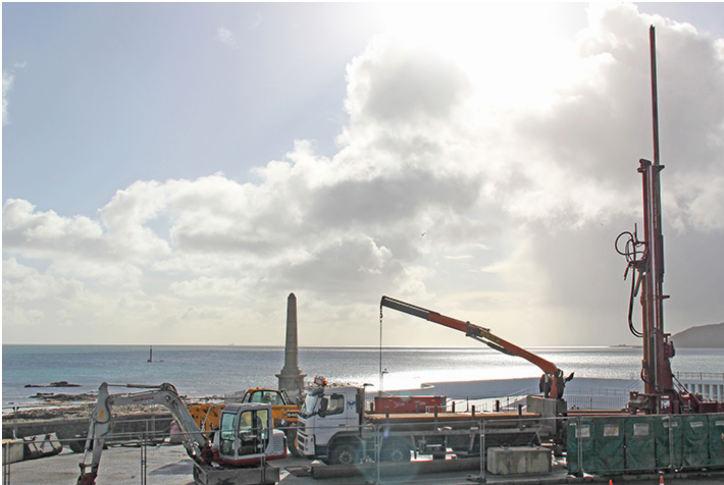
Construction of the geothermal well at Jubilee Pool
