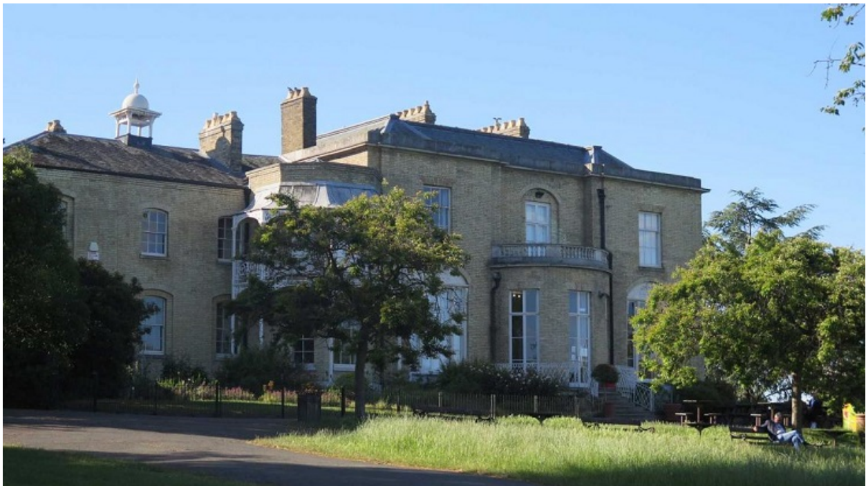
Brockwell Hall. Credit: London Borough of Lambeth/Pringle Richards Sharratt
