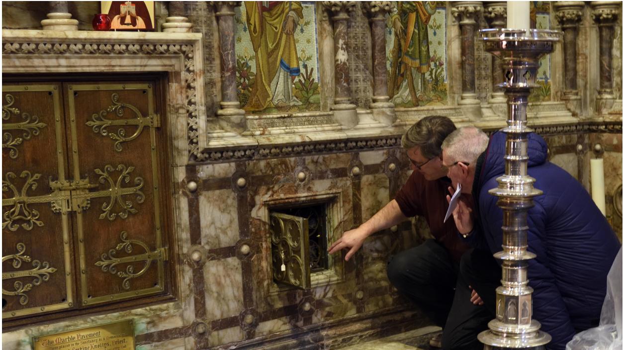
Inspecting the alcove. Credit: Mark Hourahane
