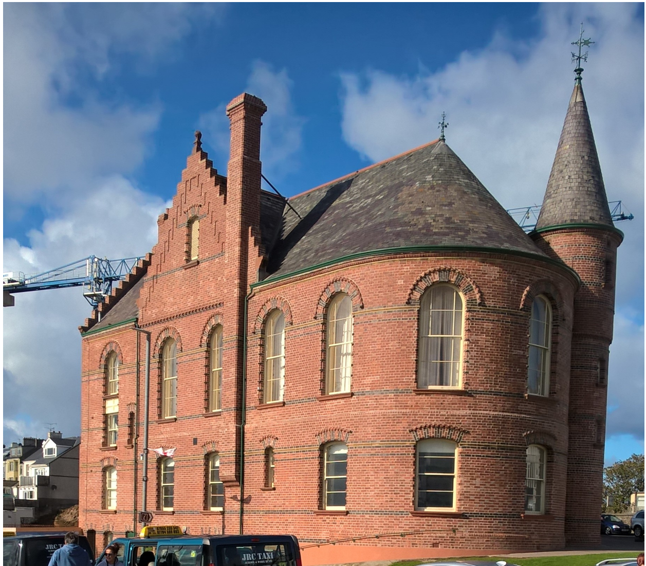
Portrush Town Hall, which was restored as a venue for community events thanks to National Lottery funding
